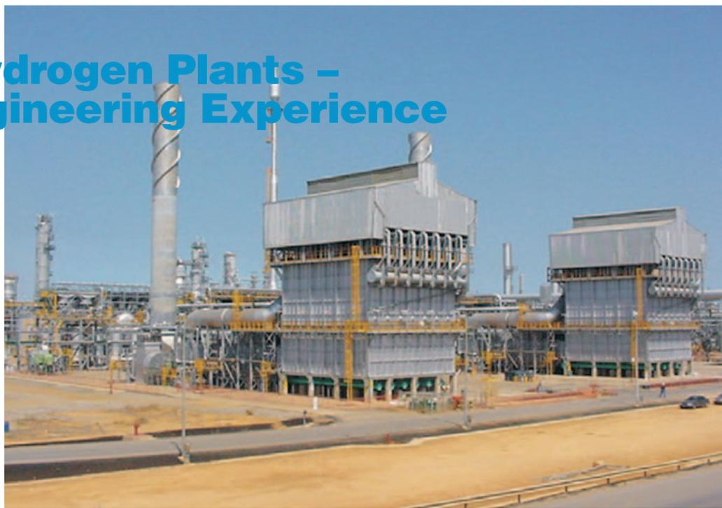
2 x 100,000 Nm<sup>3</sup>/h hydrogen manufacturing unit at the SINCOR upgrader, Venezuela
