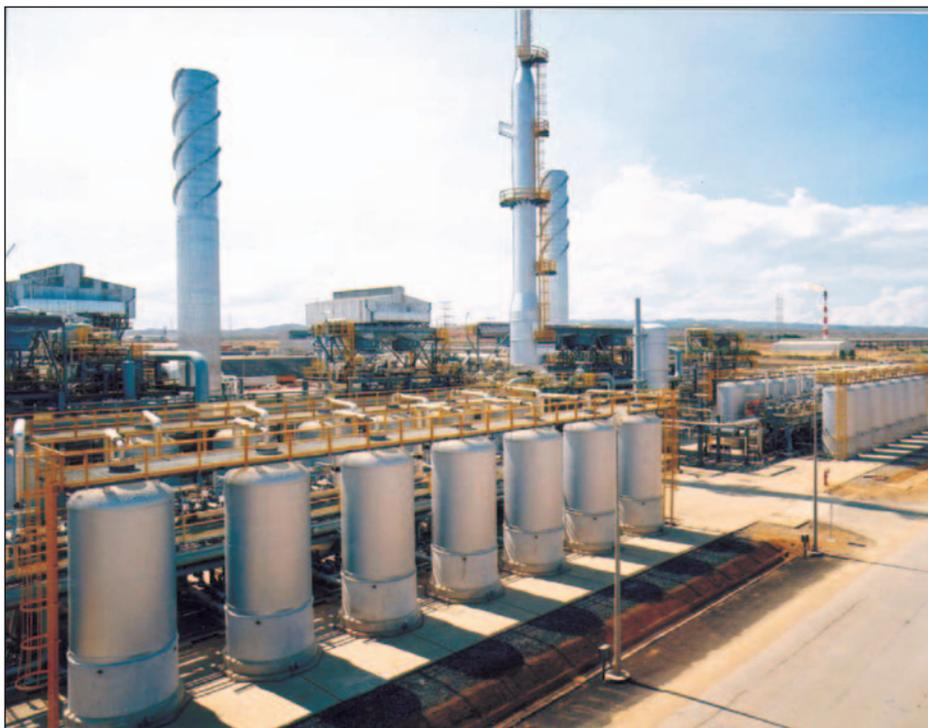
Fig. 8 Site view PSA – 14-Adsorber Polybed Units of UOP at the SINCOR upgrader
