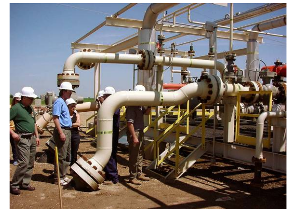
Weyburn Pipeline http://www.ptrc.ca/access/DesktopDefault.aspx
